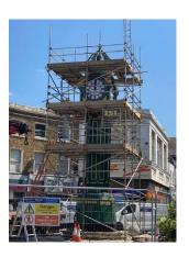
On 18<sup>th</sup> May with the tower fully in position Smith of Derby started to install the four bracket arms and new lanterns before the scaffolding was then removed. Smith of Derby also started to install the electrical cables within the tower. UK Power Networks (UKPN) were also on site to reconnect the power supply to the tower.
